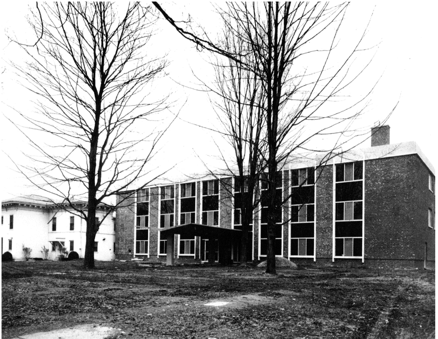
Bertrand Chaffee Hospital, before demolition of Bertrand Chaffee house, ca. 1970 (courtesy of Concord Historical Society)
