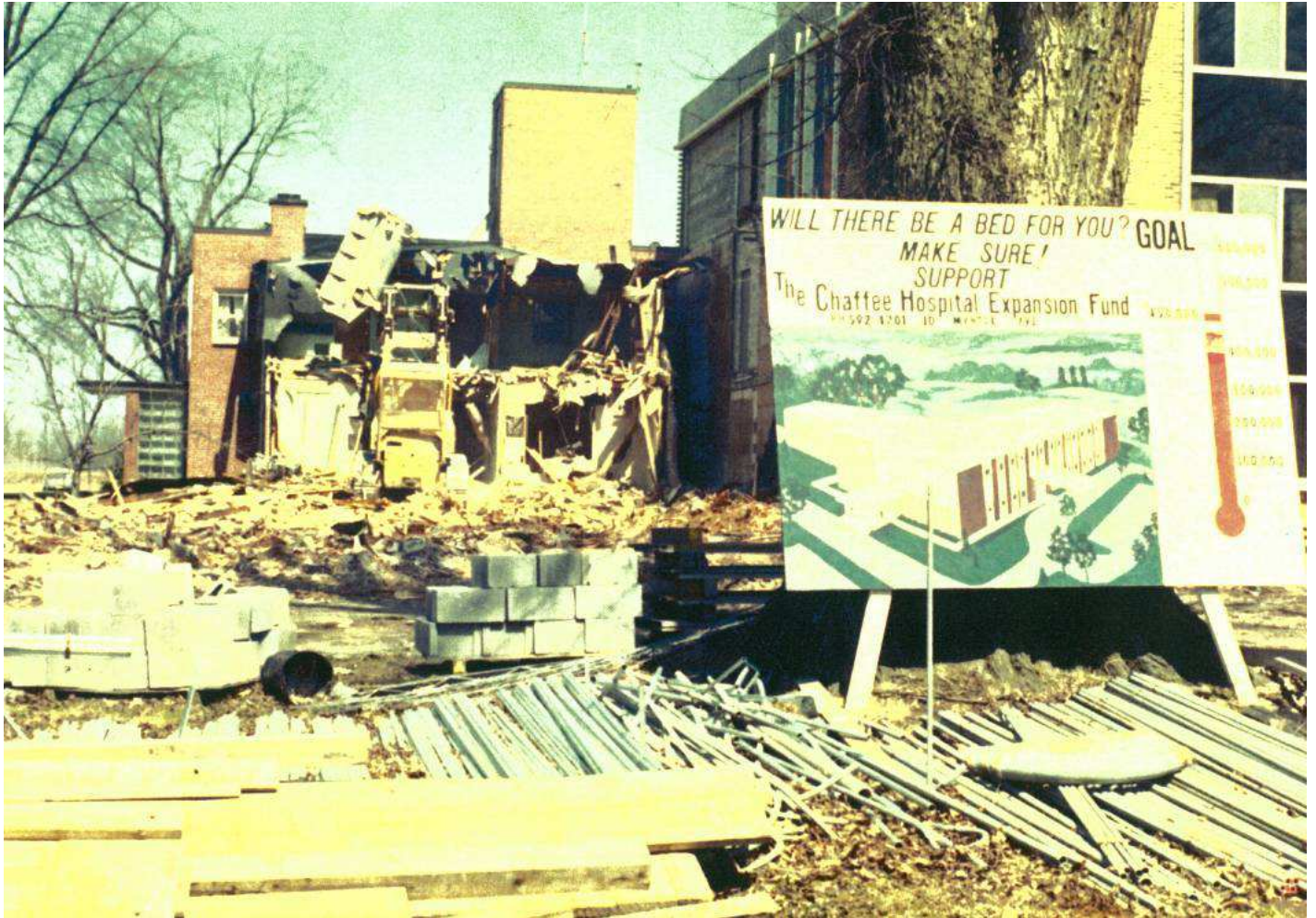
Bertrand Chaffee Hospital, Demolition of Bertrand Chaffee house, ca. 1970 (courtesy of Concord Historical Society)
