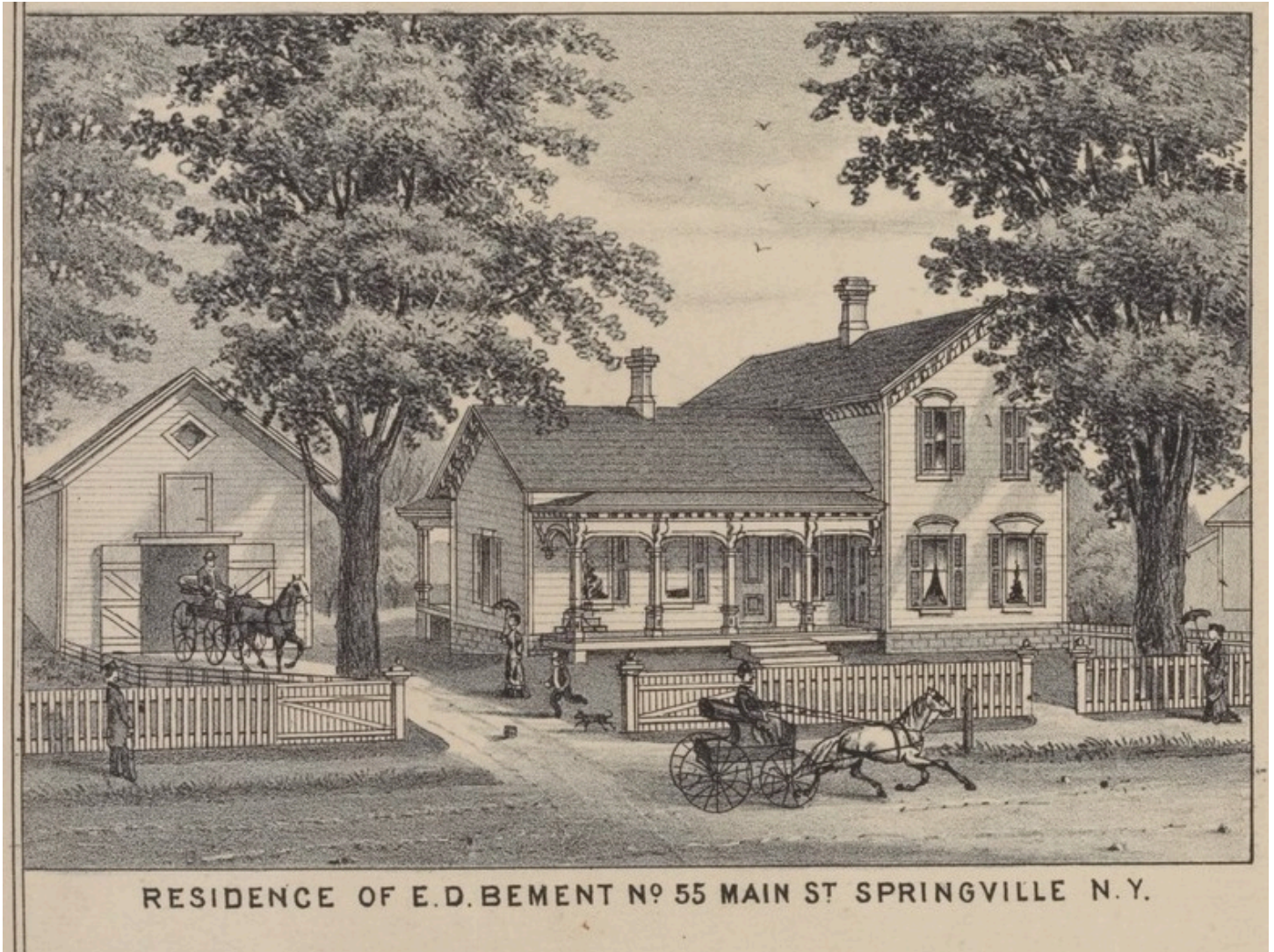
E.D. Bement House, 148 West Main Street, 1880 From the Illustrated Historical Atlas of Erie County, New York (Illustration courtesy of the New York Public Library Digital Collection)
