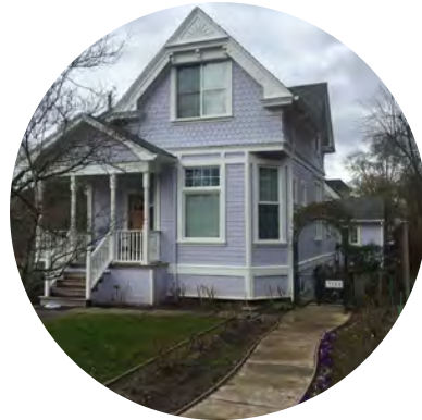
Basement Conversion to ADU
